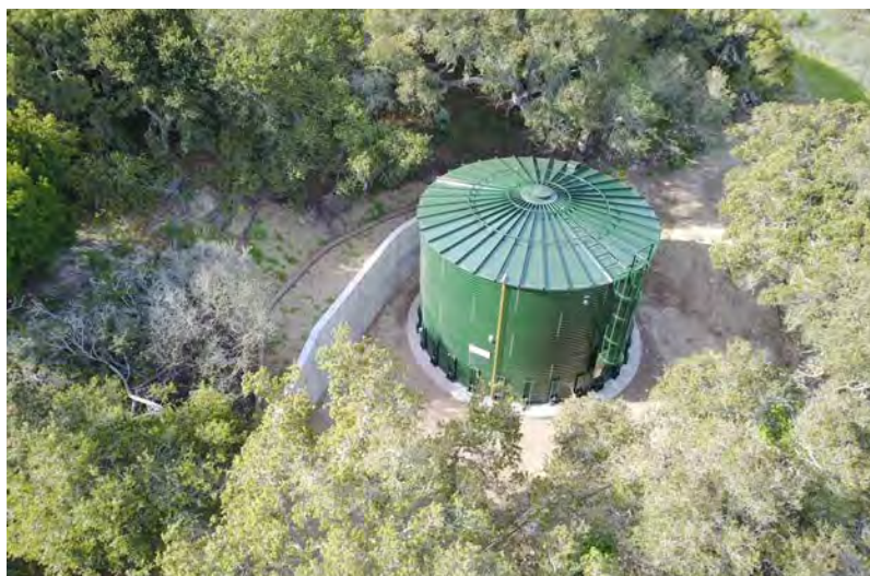
This green, corrugated steel water storage tank is what most people think about when tanks are mentioned. It’s color is intended to help it blend in with the
